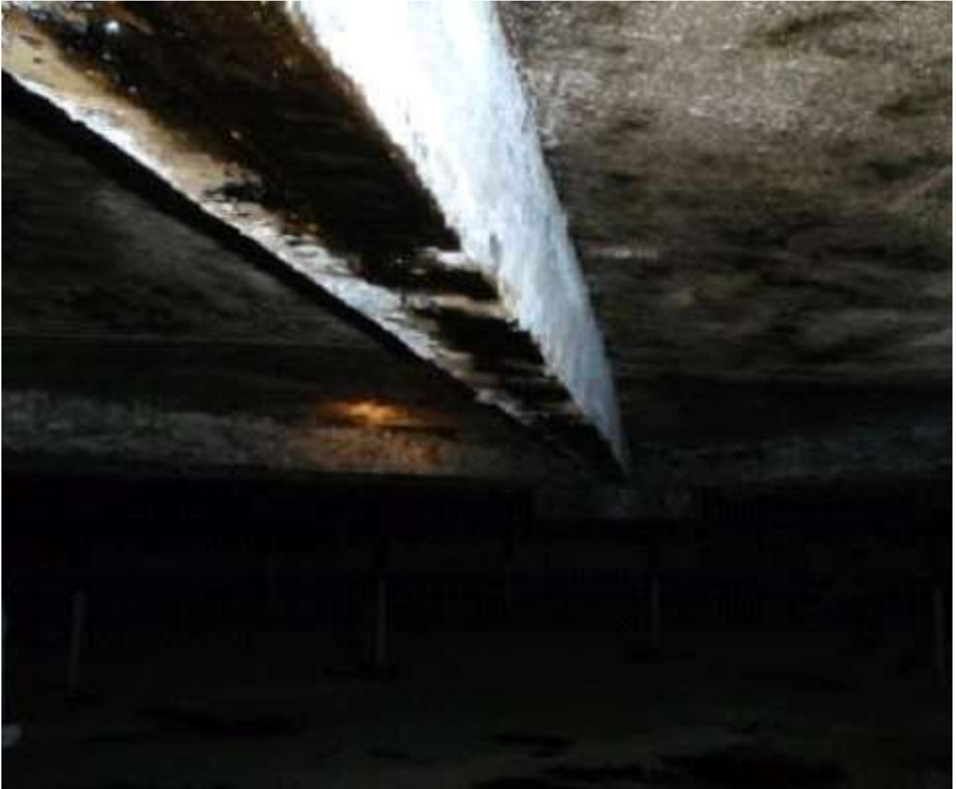
Photograph 4 of 6 CONVENTIONAL MECHANICAL CLEANING
