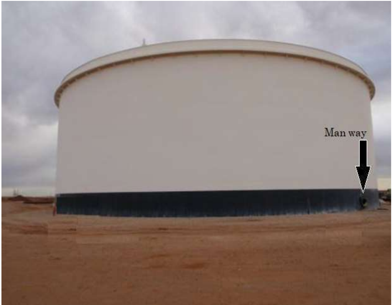
Photograph 1 of 6 PDS-660 CHEMICAL CLEANING RESULTS
