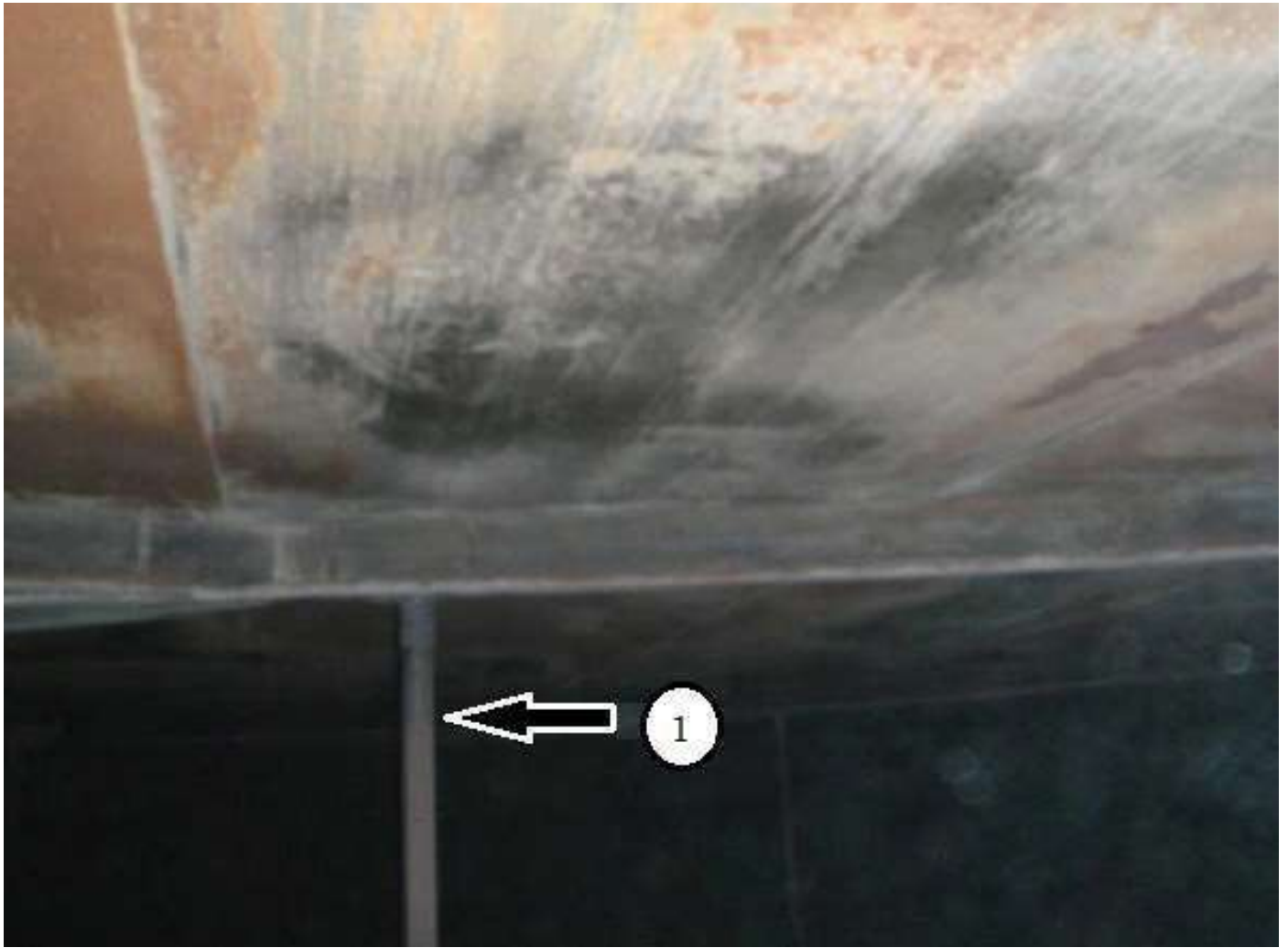
Photograph 5 of 6 PDS-660 CHEMICAL CLEANING RESULTS
