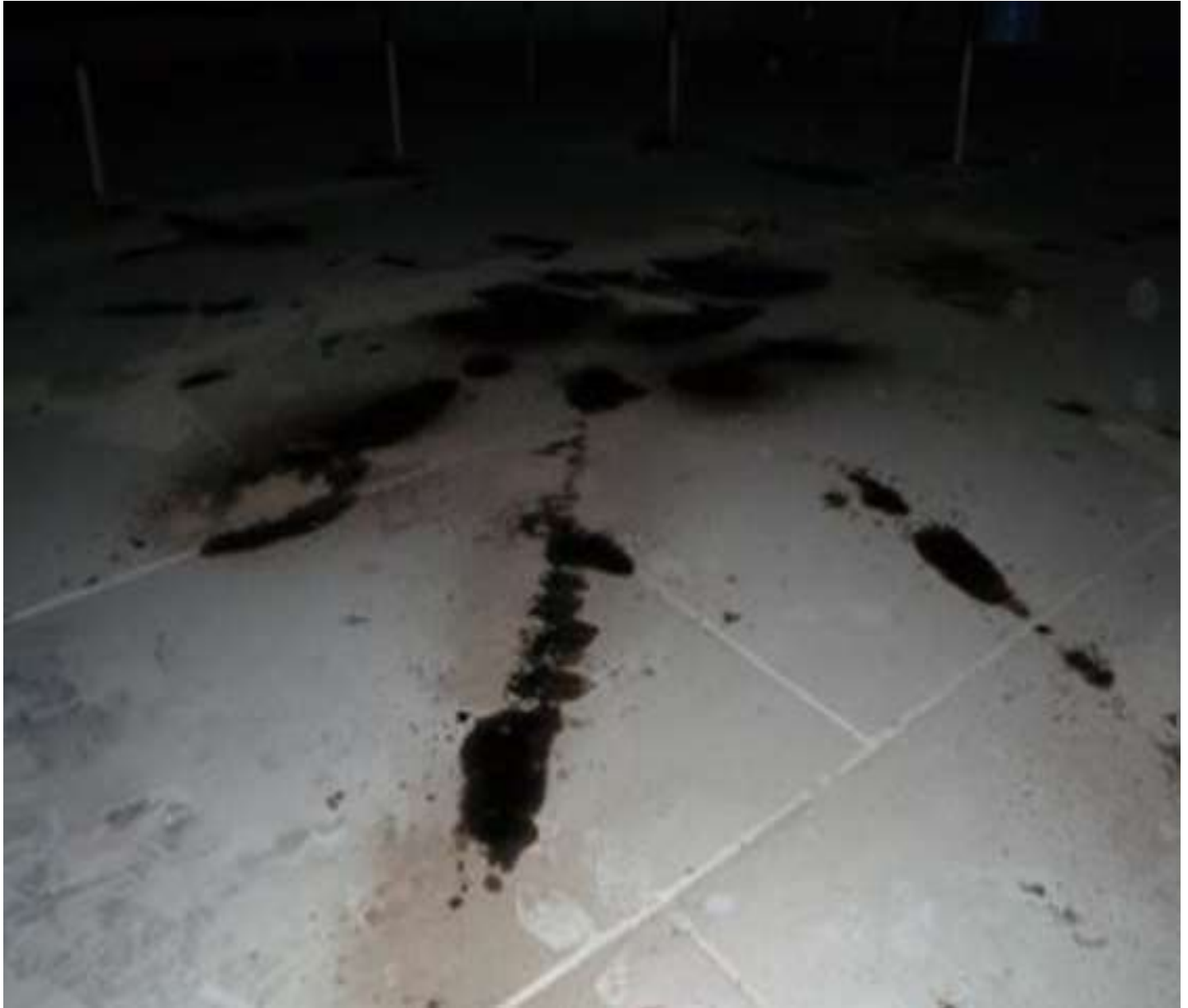
Photograph 5 of 6 CONVENTIONAL MECHANICAL CLEANING
