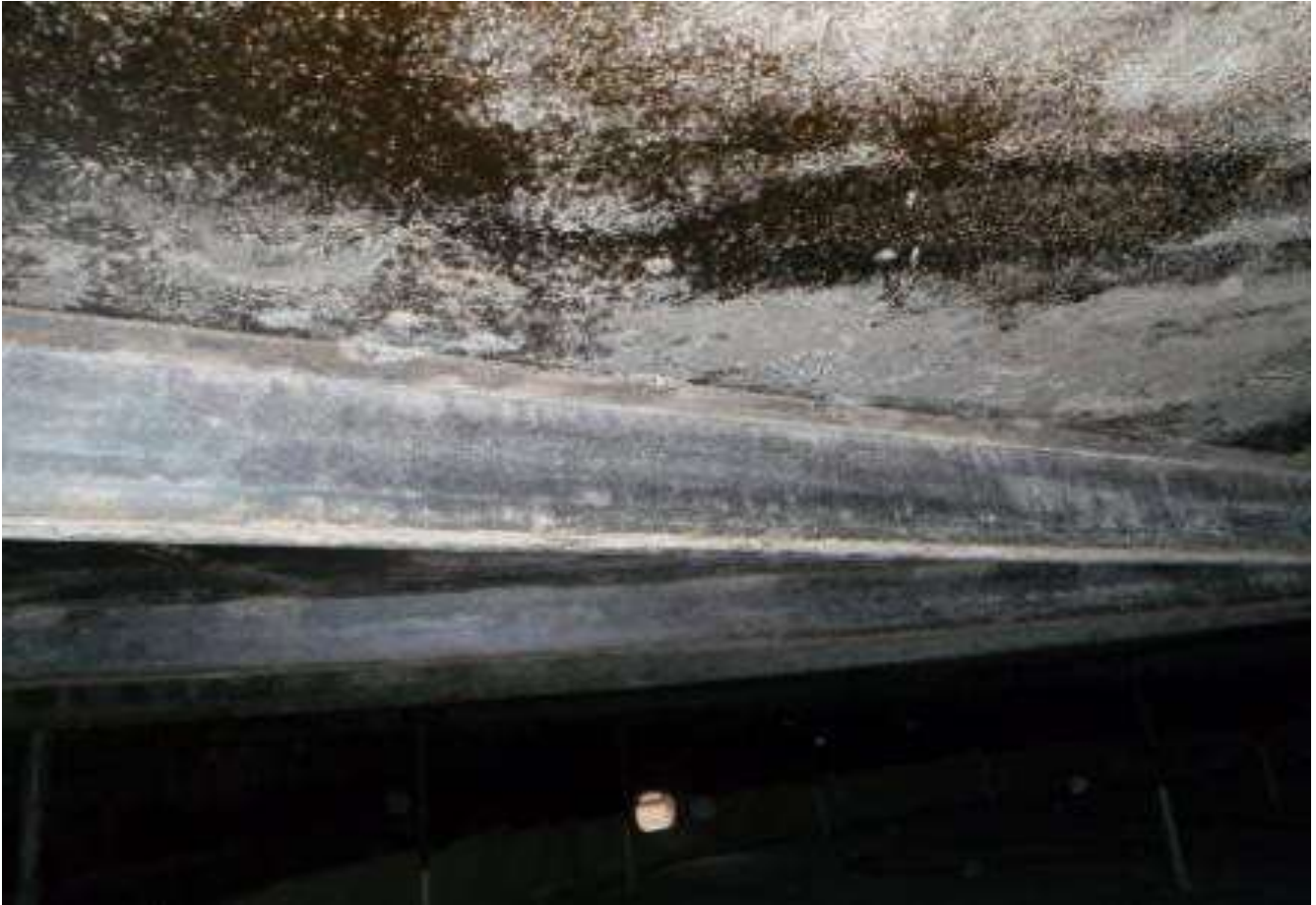
Photograph 1 of 6 CONVENTIONAL MECHANICAL CLEANING
