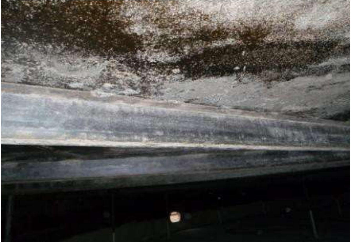
Photograph 1 of 6 CONVENTIONAL MECHANICAL CLEANING
